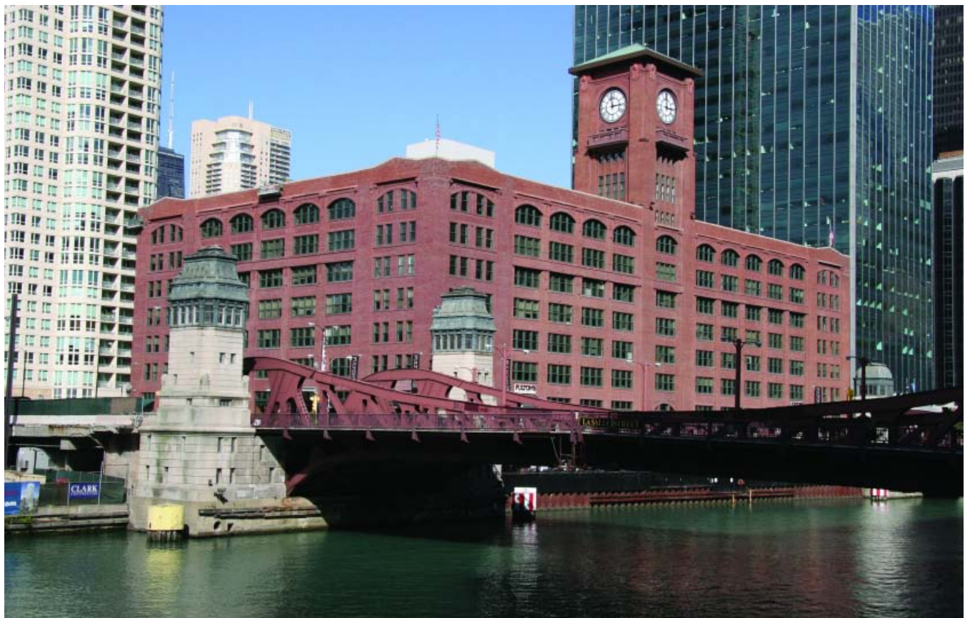
Historic Reid Murdoch Center. (Photos by Mark Samuels.)
