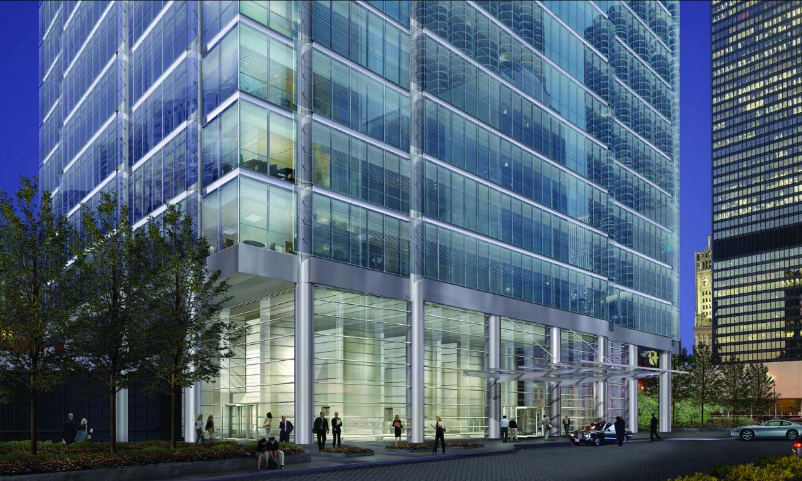
A new 45-story office tower will feature state-of-the-art technology and a variety of tenant amenities including an on-site health club and dining facilities.
