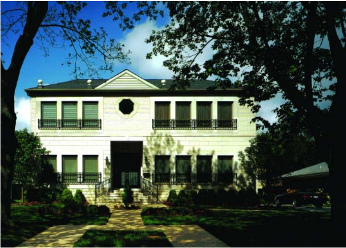
Classic simplicity and clean, spare lines distinguish the Lincolnwood, Ill., home. Decorative ironwork and metal window frames meld fluidly with the monochromatic color scheme. The formal landscape plan creates an outstanding residence whose beauty is timeless.
