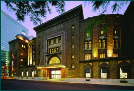
The American Institute of Architects honored Daniel P. Coffey & Associates, Ltd. with its Distinguished Building Award for the firm's work with Friedman Properties, Ltd. on the redevelopment of Medinah Temple. (Photo by James Steinkamp)
